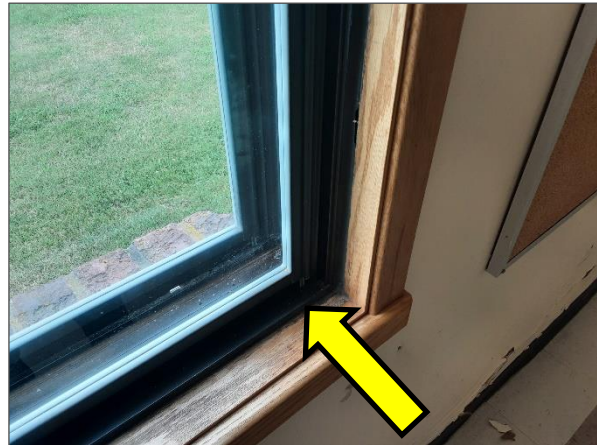
Non-asbestos dark brown caulking.
