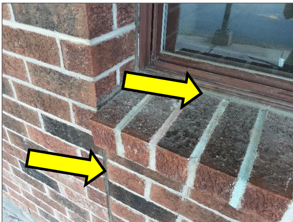
Non-asbestos light brown caulking.
