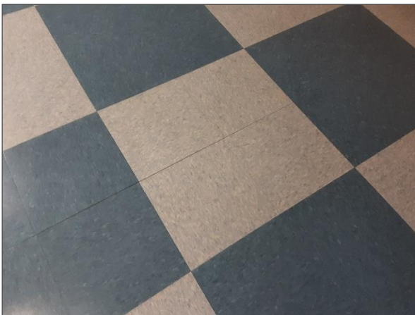
Non-asbestos blue and light blue vinyl floor tiles with fleck.
