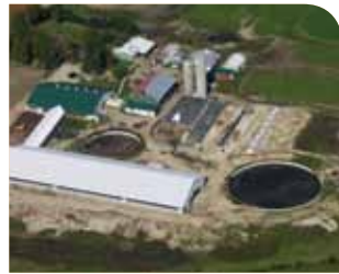
Barns, manure storages and other associated buildings and structures
